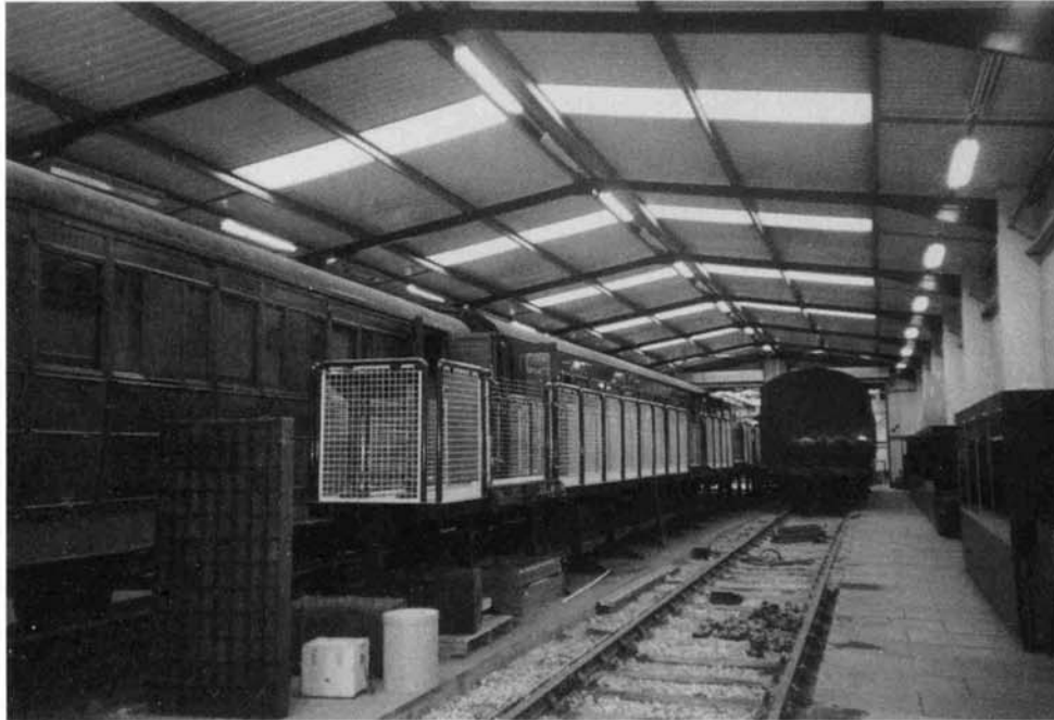
The new central walkway - a view possible only when coaches are out of the Museum
