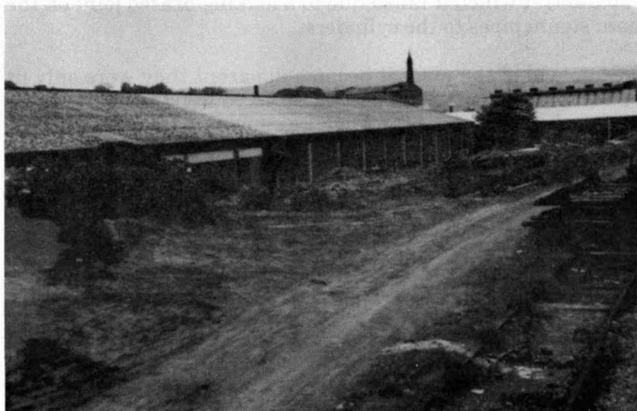
Foundations of Ingrow Carriage Shed, Spring 1988
